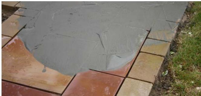
Pour the Jointing Mortar onto the pre-soaked paved area. Using a squeegee, work the slurry into the joints.
