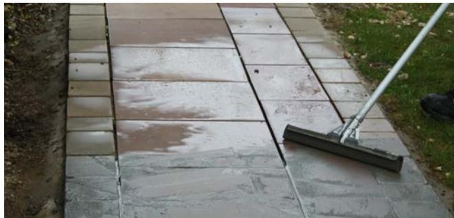
Using the rubber squeegee remove as much mortar as possible from the paved surface, whilst ensuring that all joints remain filled. Don't let the residue on the surface go matt, keep the area moist.
