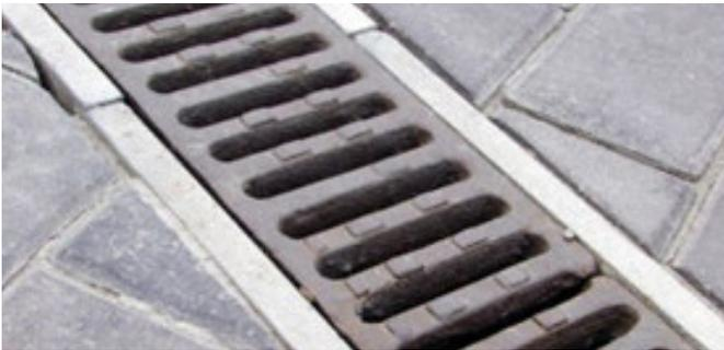
Cover any drains to prevent any mortar from getting into them, you can use plastic bags and duct tape.
