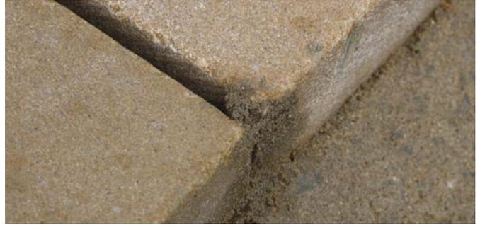
Blank off any open ended joints with modelling clay, or a firm mortar or sand.
