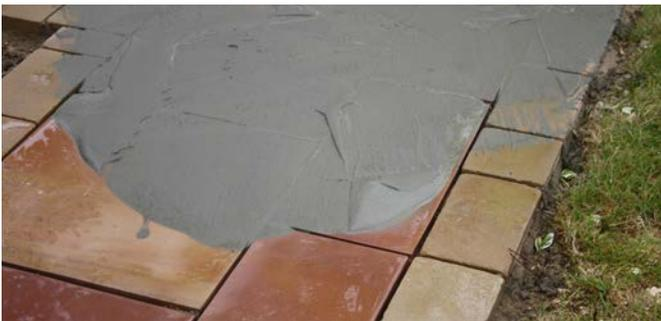
Pour the Jointing Mortar onto the pre-soaked paved area. Using a squeegee, work the slurry into the joints.
