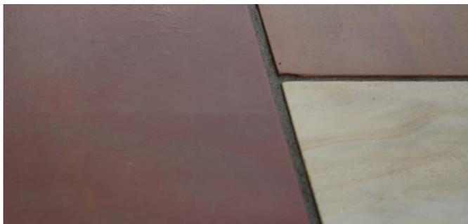
Repeat the last step until the water that runs off the surface of the paving is completely clean and clear - indicating that there is no mortar residue remaining on the surface of the paved area.
