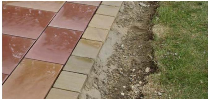
Plan the direction that you wish to brush off the excess mortar and ensure it has somewhere safe and practical to go – as any residue will set hard, could stain and cause problems if it goes into drains or similar.
