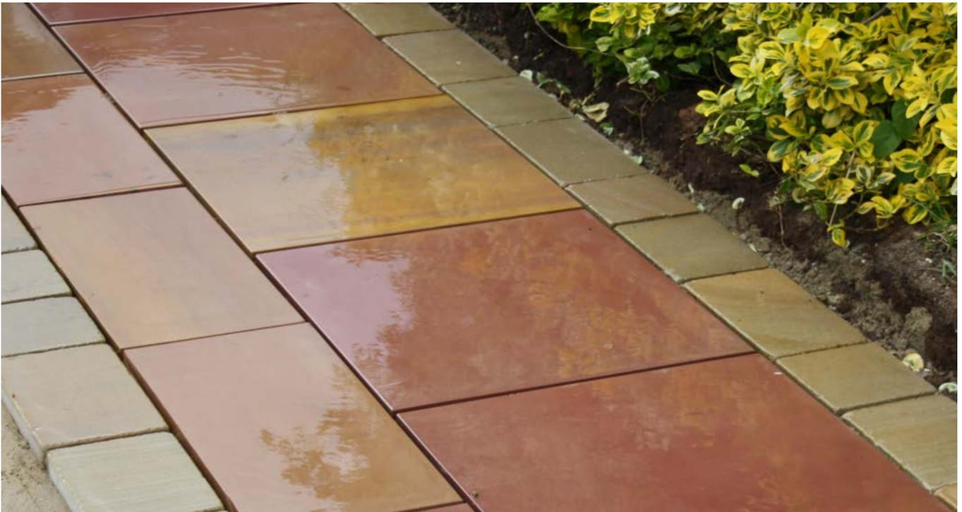
Thoroughly saturate the paving and joints before application, any standing water should be brushed away.
