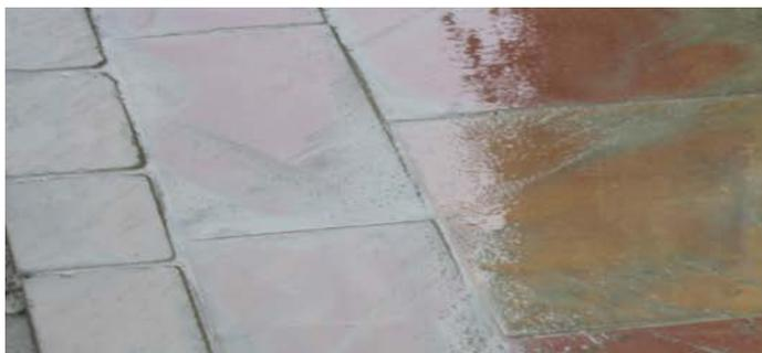
While waiting for the Jointing Mortar to firm up, which takes approximately 15 minutes at 20°C surface and air temperature, the area and joints must be kept wet. Mist water on the surface using a low-pressure jet wash, pointing the lance along or upwards from the paving never directly on to it. Take care not to wash out the material in the joints.
