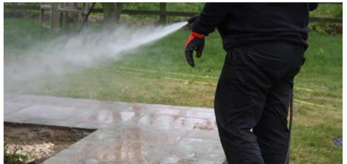
Ensure the paved area is kept completely wet throughout, until the entire area has been jointed and the joints have set firm. We suggest you mist the water on to the surface using a low pressure jet wash, pointing the lance along or upwards from the paving, never directly onto it.
